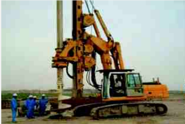
Concrete bore pilling and steel drilled steel I-section pilling
