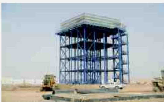
Elevated water storage tanks 25 m high and capacity of 2250 m 3 storage volume
