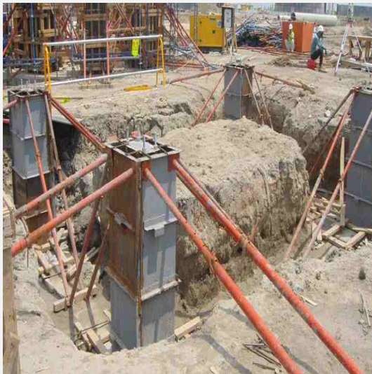
Metal form work for pipe rack pedestals
