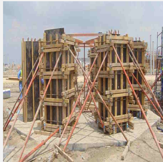
Form Work for Heater foundation pedestals
