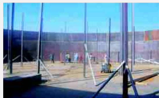
Elevated water storage tanks 25 m high and capacity of 2250 m 3 storage volume
