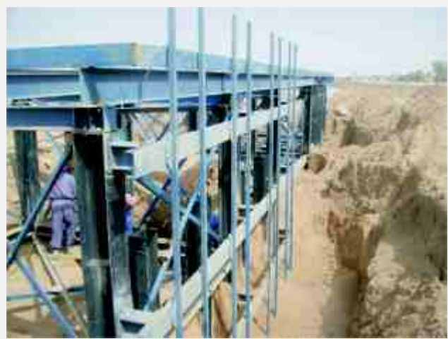
Concrete bore pilling and steel drilled steel I-section pilling
