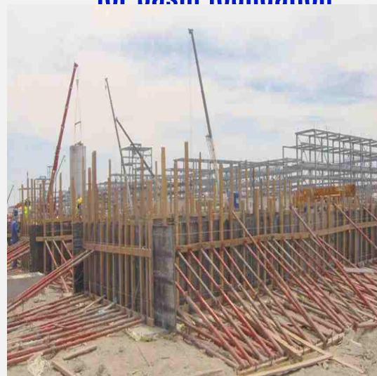
Reinforcement and form work for hasin foundation
