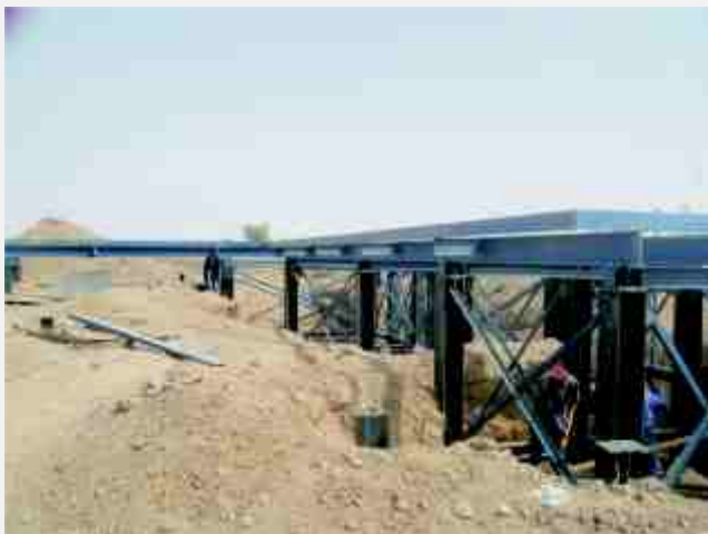
Concrete bore pilling and steel drilled steel I-section pilling
